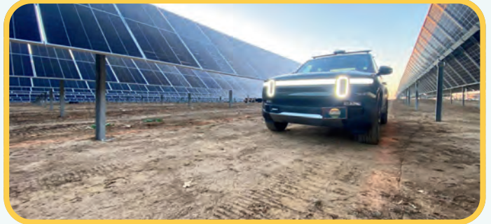
One of Village Solar Co.'s Rivian electric vehicles in a solar field.
