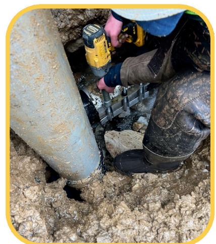
Village employee Lucas Valley installing a repair band at a recent water main break.
